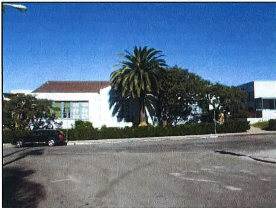
Figure 13: Front (south) façade of the Main Building of North School presenting the exterior façade that is a result of the repairs and rehabilitation in 1934. View looking north.
