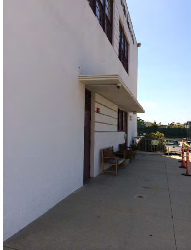
Figure 4 – North Exterior Wall Looking West
