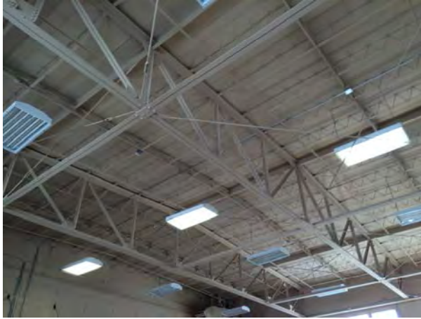
Figure 1 – Steel Roof Trusses in Gymnasium
