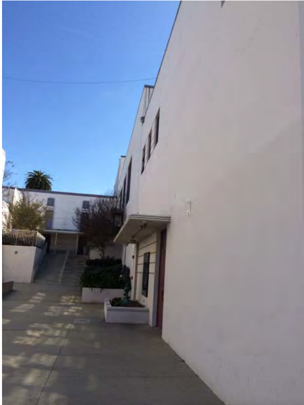
Figure 3 – North Exterior Wall Looking East
