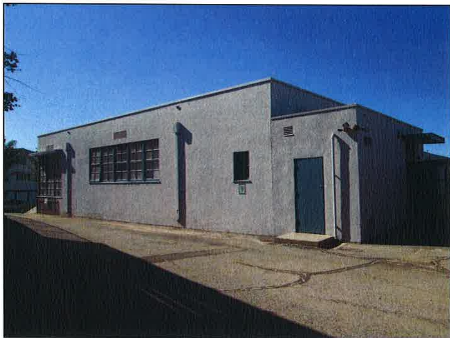
1939 Kidergarten Building, view looking southwest. November 2015.
