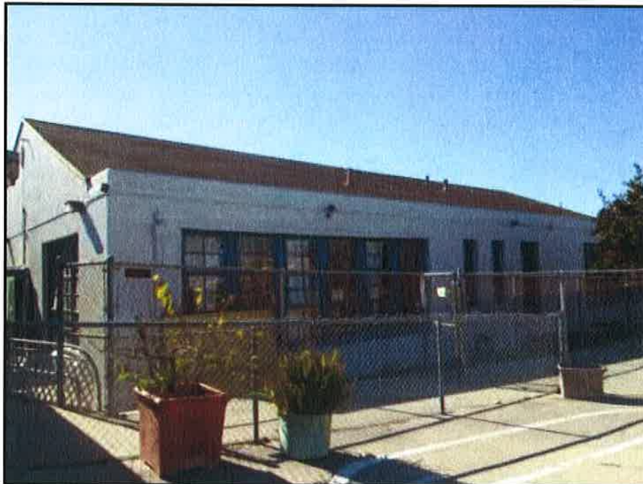
Figure 14: Rear (north) façade of the main North School building. Its gable roof is easily viewed from this direction. View looking southwest.
