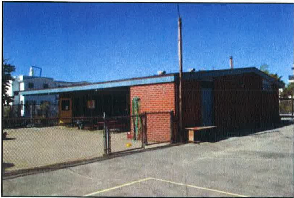
Figure 18: 1958 Kindergarten building. View looking northwest.
