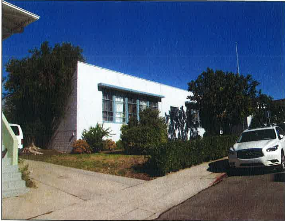
1939 Classroom Building, view looking northeast. November 2015.
