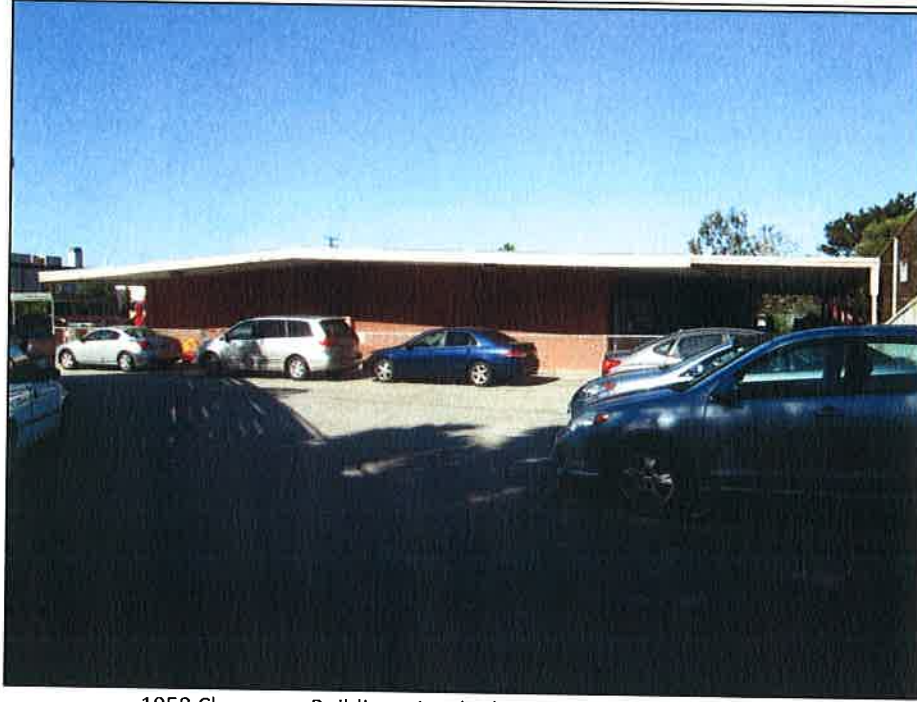
1958 Classroom Building, view looking north. November 2015.
