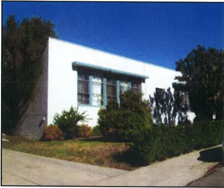
Figure 17: The 1939 Classroom building. View looking northeast.
