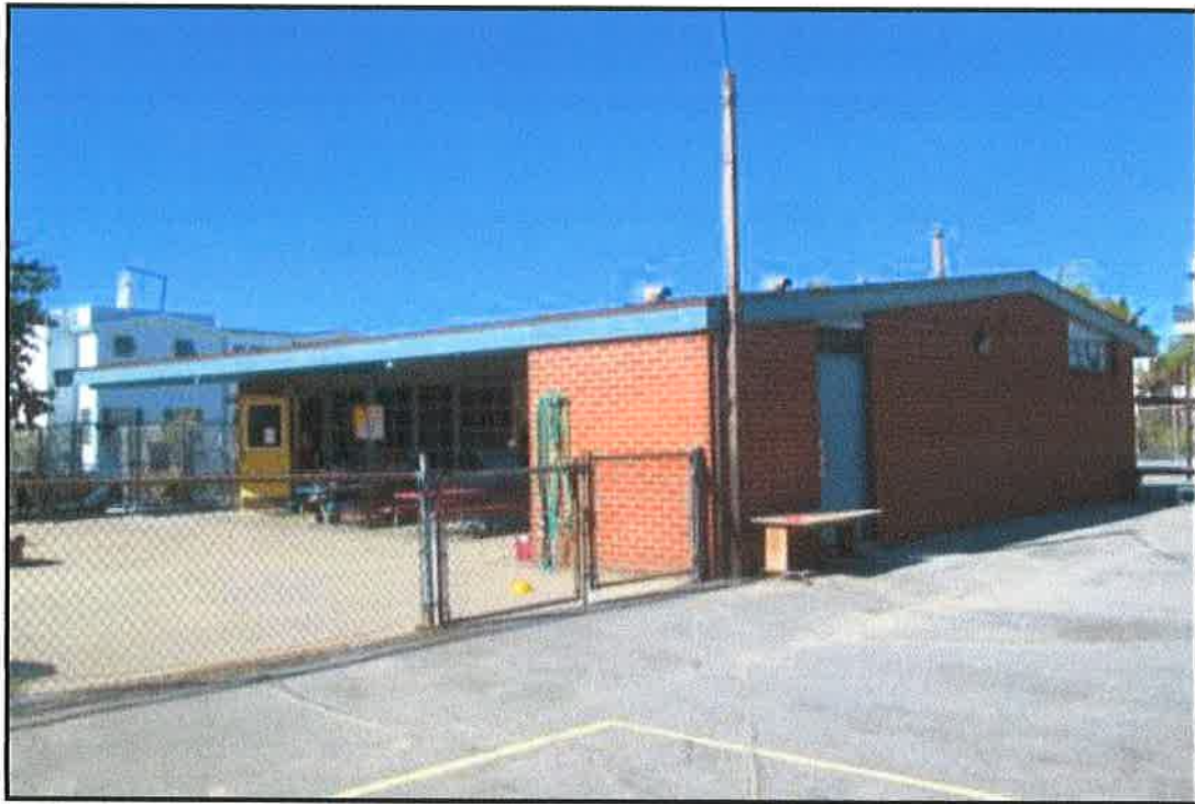
Figure 18: 1958 Kindergarten building. View looking northwest.
