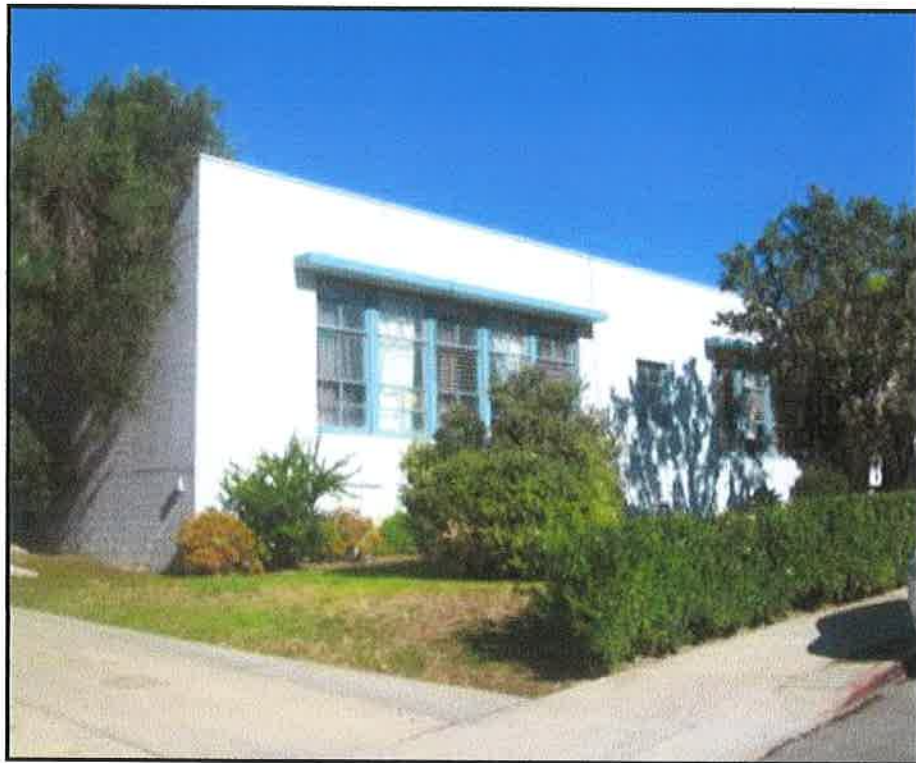
Figure 15: The 1939 Classroom building. View looking northeast.
