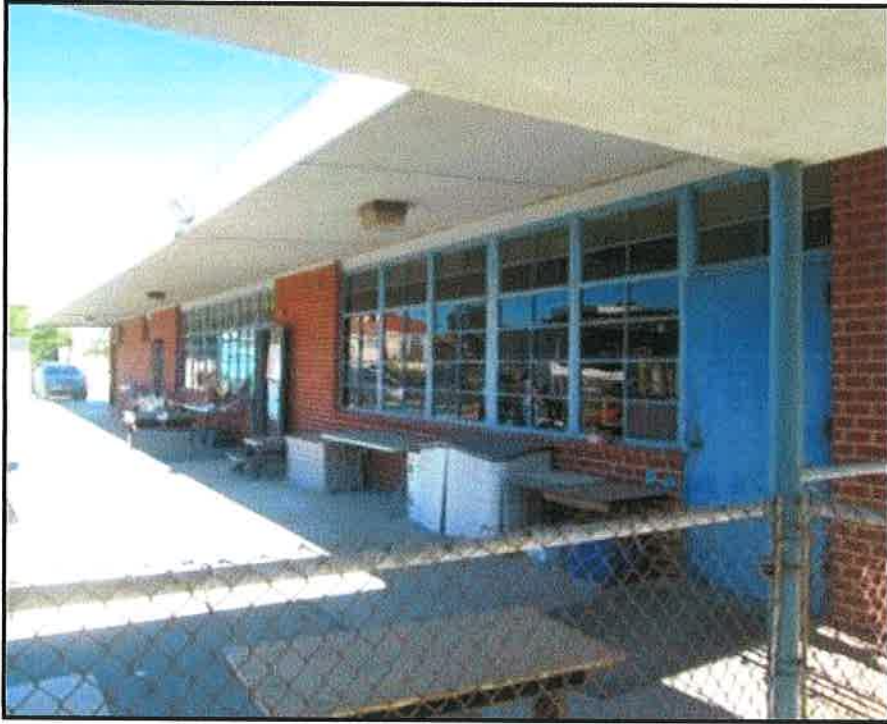
Figure 16: West façade of the 1958 Classroom building facing the inner courtyard. View looking north.
