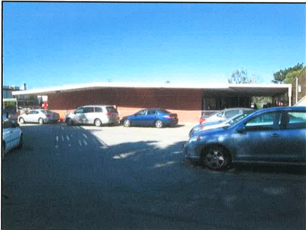
Figure 17: South elevation of the 1958 Classroom building. View looking north.
