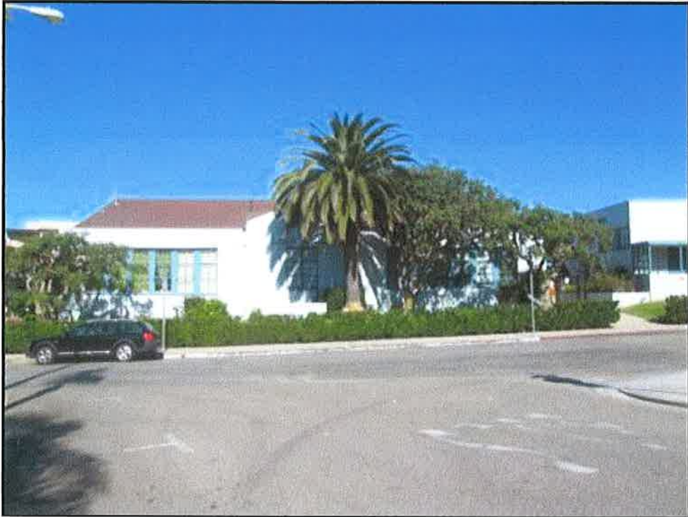
Figure 11: Front (south) façade main North School building, as reconstructed in 1935 after the Long Beach earthquake. View looking north.
